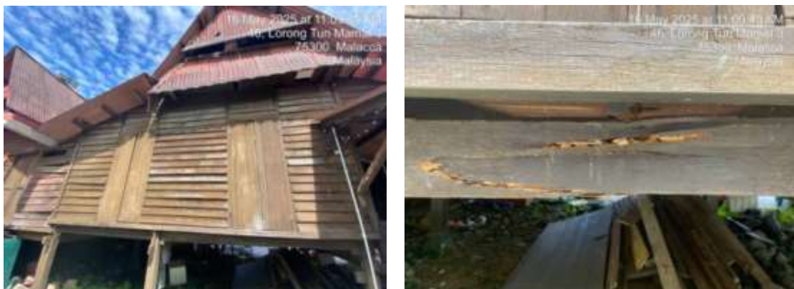
Figure 13: The decay in floor boards and joist impacted the structural condition of house 3
