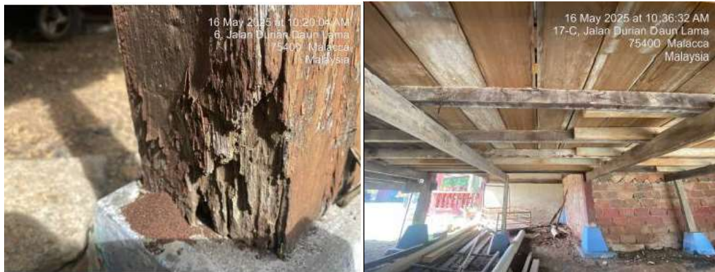
Figure 14: Termites attack at the column and floor boards
