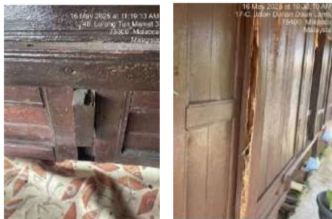
Figure 11: The internal condition of the house showing column and joins decay
