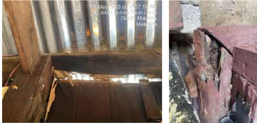
Figure 12: The structural decay of roof beam (left) and column (right) is the major defect for House 2
