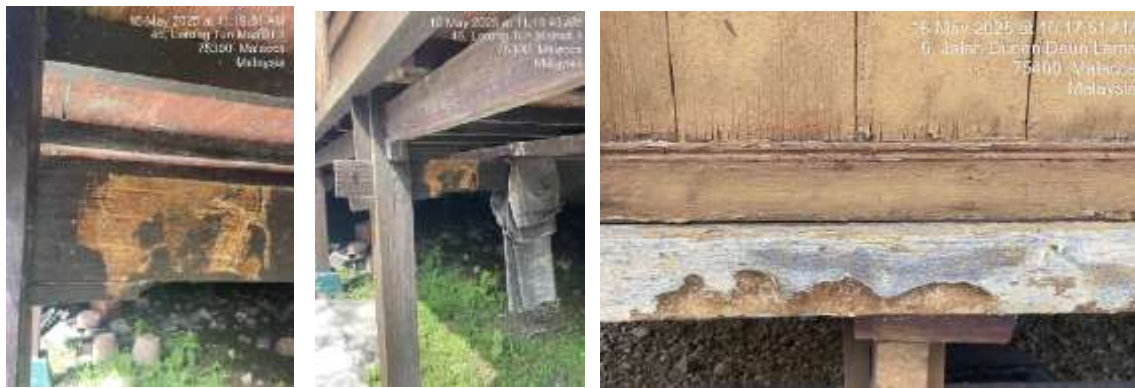
Figure 10: The termites attack and decaying external structure of House 1
