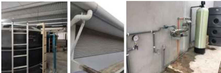
Figure 4.8: Rainwater Harvesting System with Filtration in UM
